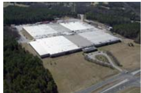
Springs Katherine Plant
